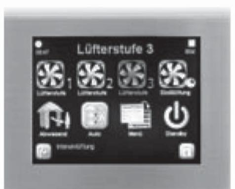
The fresh air system can be left on "auto" but you can press the boost button during cooking or if the bathroom is steamy. If you go away during the winter leave it on the lowest speed '1' to ensure warm fresh air on your return.
