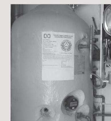
In summer the whole tank is heated up by the sun when it shines on the solar panels on the roof. In winter the sun heats the bottom half of the tank and the boiler heats up the top so you always have hot water even when there is no sun.
