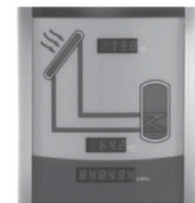
Hot water should always be ready - the tank is very well insulated so it won't cool down overnight. You can see how much the sun has heated has the bottom half of the tank by looking at the display. In winter most of the hot water will come from the boiler.
